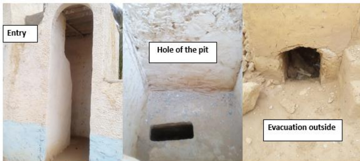
Figure 3: dry toilets architecture in the M'zab valley
