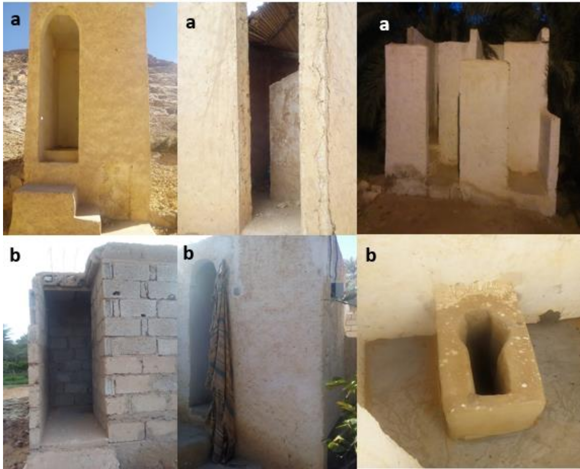
Figure 4: private and public dry toilets in M'zab Valley (a: private; b public)
