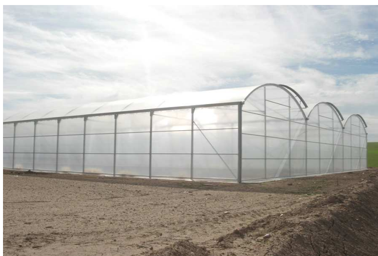
Fig. 30 – Serres multi chapelles couvertes de filet insect proof
