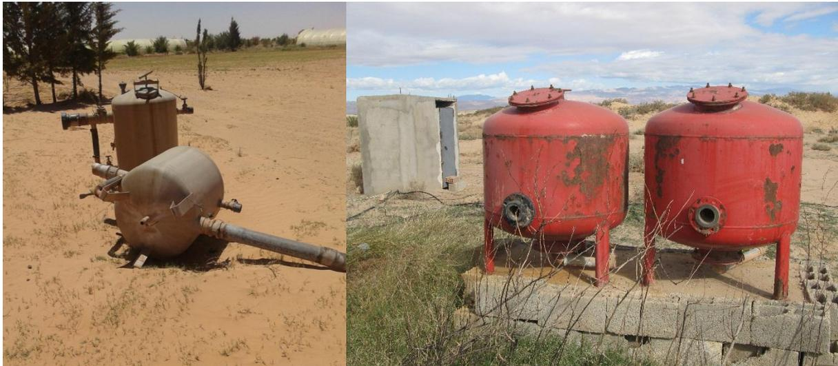
**Figure 22. Abandoned filter systems from the subsidised irrigation systems in Biskra**
