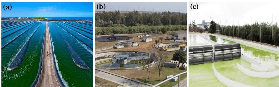
Figure I.2: Photos of open ponds for algae farming: (a) raceway ponds at Cyanotech algae farm (Hawaii, USA), (b) circular ponds at Aqualia All Gas (Sevilla, Spain), (c) paddle wheel ponds at Biorizon Biotech (Almeria, Spain).
